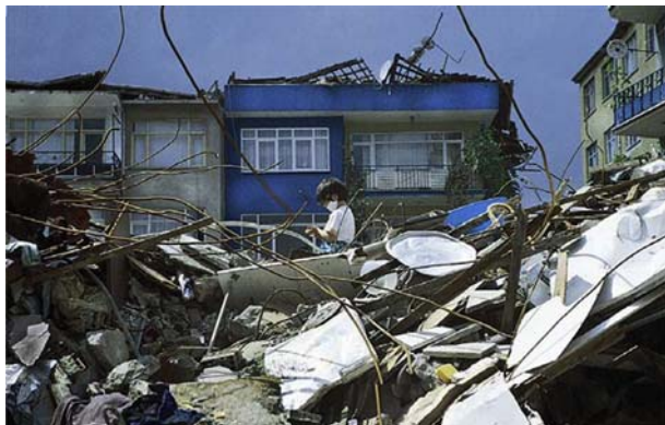
Figure 9. Turkey earthquake (1998). (Courtesy of Dr Briggs.)
