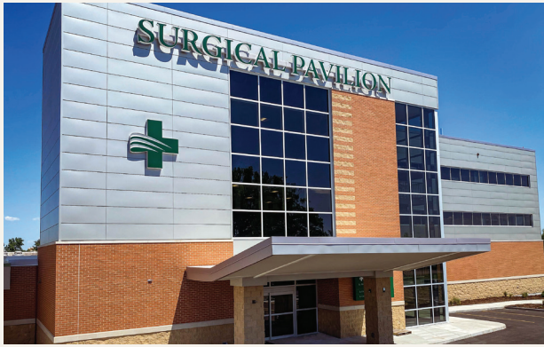
Fairfield Memorial Hospital Surgical Pavilion
