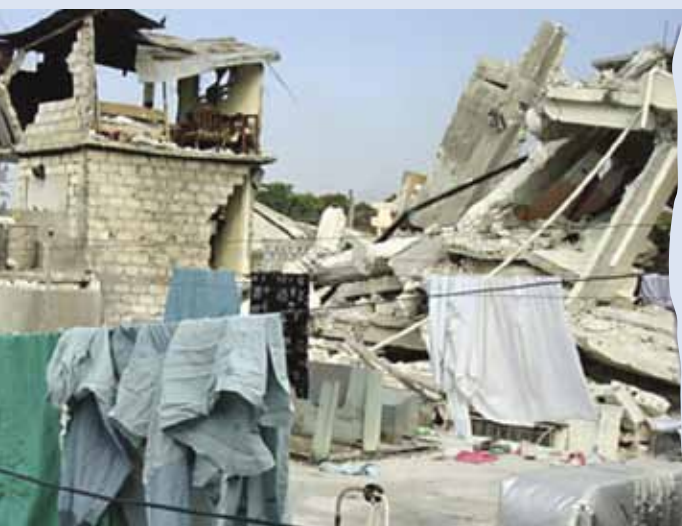
Scenes of post-earthquake destruction in Haiti. In the bottom photo of the collapsed pediatric hospital, a bed can be seen near the edge of the remaining tower at left.
