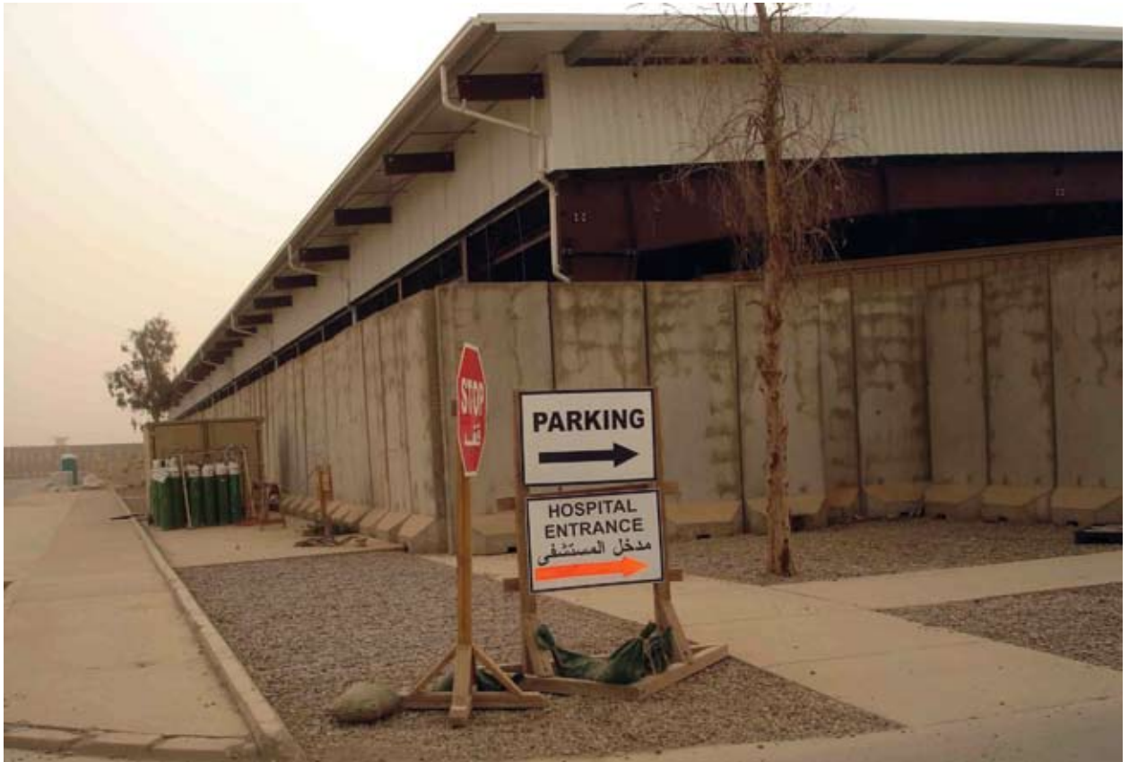
Entrance to the emergency department at the 332nd.
