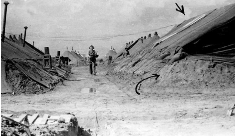
The OR, dug in with three-foot revetments and hail roof after the shelling on March 22, 1944. The top arrow points to the OR tent, which had a two-inch gum wood roof for hail protection. The lower arrow points to the revetment. Pictured is Lt. Liz Davis, “an especially fine nurse.”
