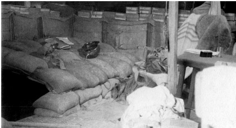
Dr. Tipton's bunk in the fourth foxhole after engineers dug the soldiers in, better and deeper, with revetments and sandbags on the roof to stop the bullet and shell-fragment hail. A general told the doctors, "You're in a fool's paradise."
