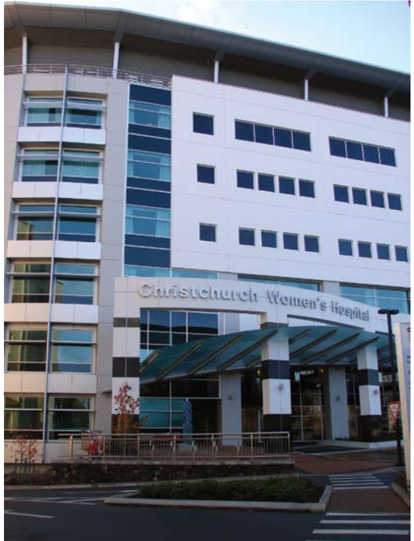
The entrance of Christchurch Women's Hospital in Christchurch, New Zealand.
