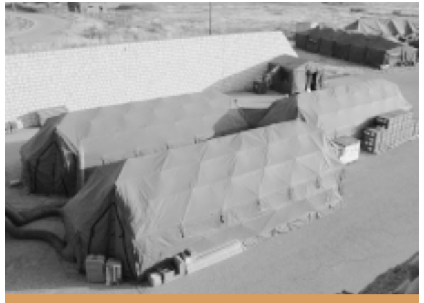
7. Three DRASH tents that comprise the 250th FST. The apical tent on the far right is the ATLS/pre-op tent; the two to the left are the operating room and SICU/post-op tents.
